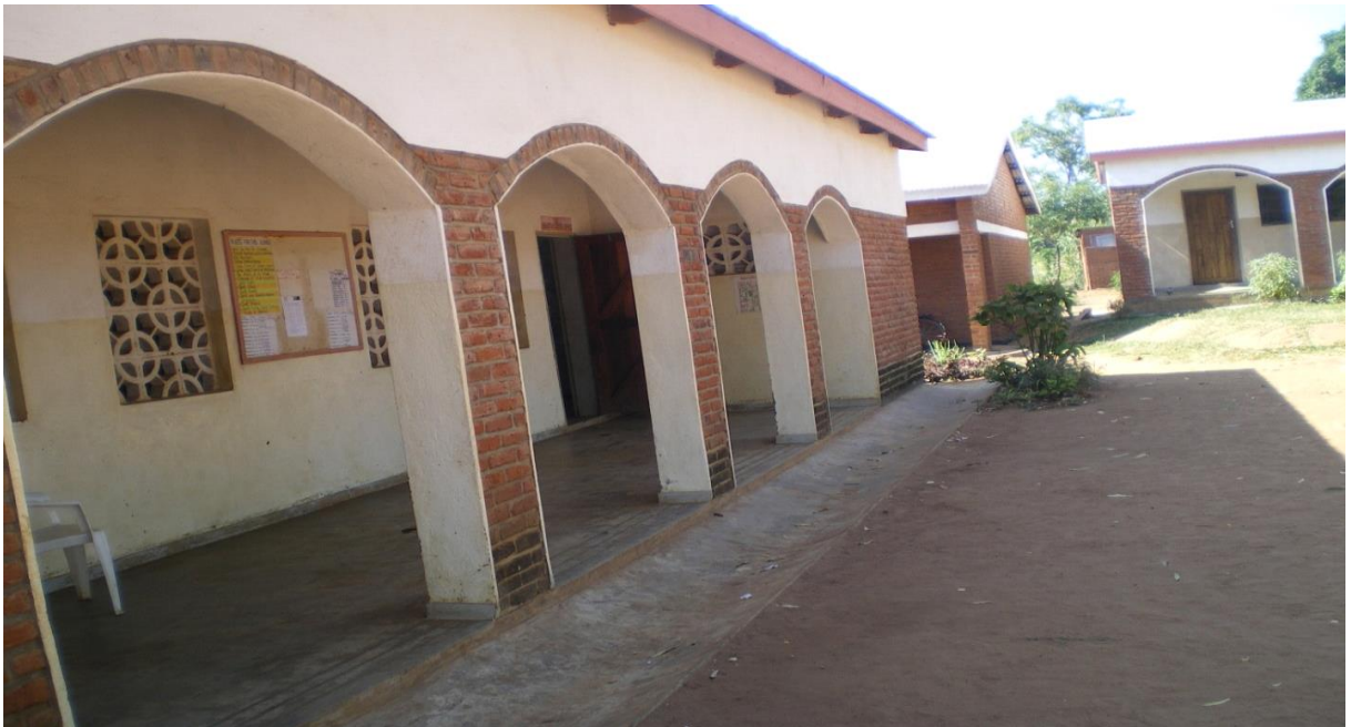
Figure 9: Classroom blocks with deep gutters
